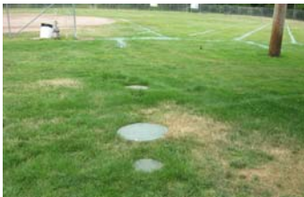
Existing Septic Drain Field
