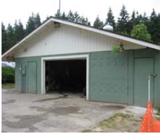
40,000 gallon cistern for irrigation water is beneath the north end of restroom / concession building.
